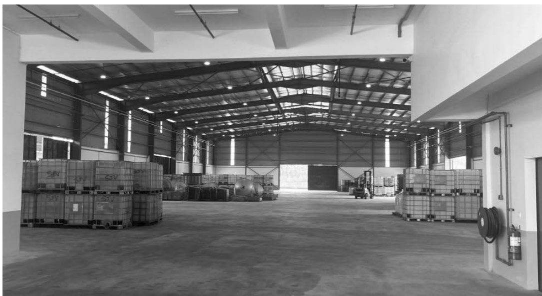
The completed warehouse at PLO 321 Facility
